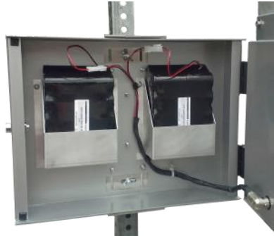
Field replacement of batteries
