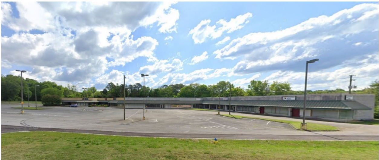
Southgate Shopping Center sits mostly vacant, Google Street View image, May 2021
