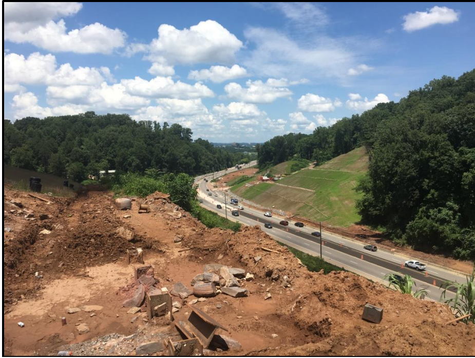
From atop of Wall 8 looking north towards Knoxville
