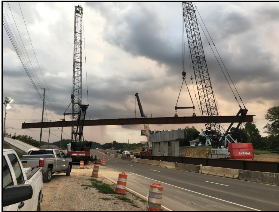
Setting Bridge #1 beams
