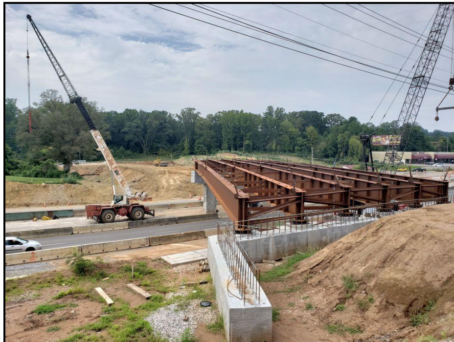
Bridge #1 with beams across span #2 set
